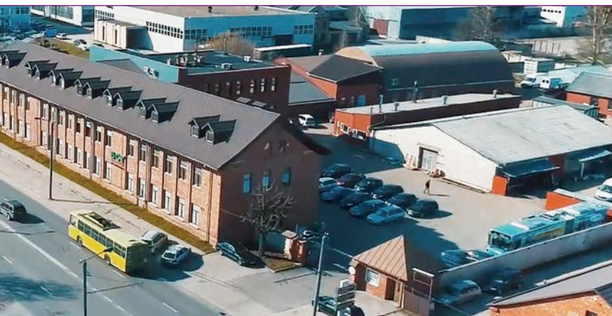
Baltec CNC Technologies company headquarters in Kaunas
